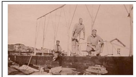
Left to right: Bill, Alan and Hughie; drilling the keel logs by hand auger
